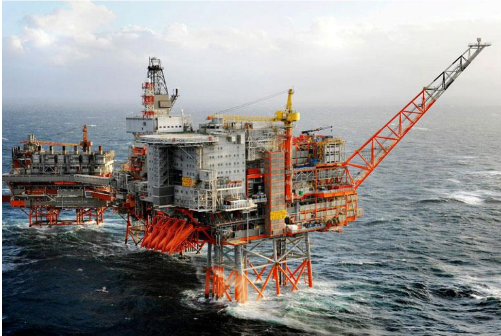
Photo 9 - Plateforme Valhall de BP (Bayards Offshore Structures, n.d.)
